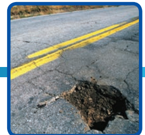
POTHoles/DAMAGED PAVEMENT
