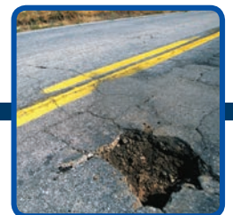
POTHoles/DAMAGED PAVEMENT
